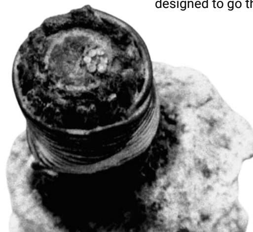
Figure 16. Damaged cable, a cross-section of the original cable showing a failure point.
